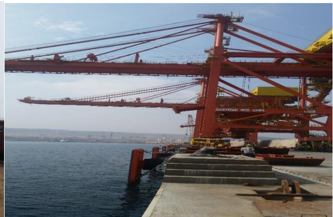
Photo 3. Docking dock with 02 gantries
